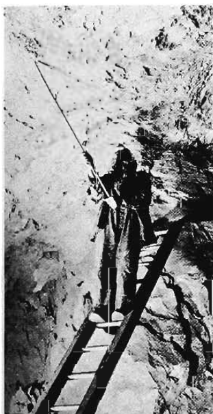
A MINER bars down loose iron ore in the underground mine at Soudan, about 1936.
