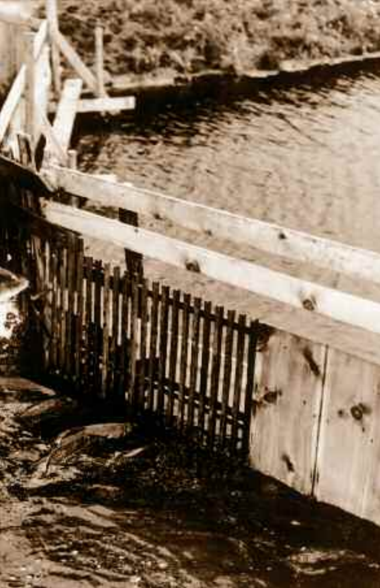
Fish trap blocking the passage of jumping carp on Six Mile Creek near Lake Minnetonka, 1965
