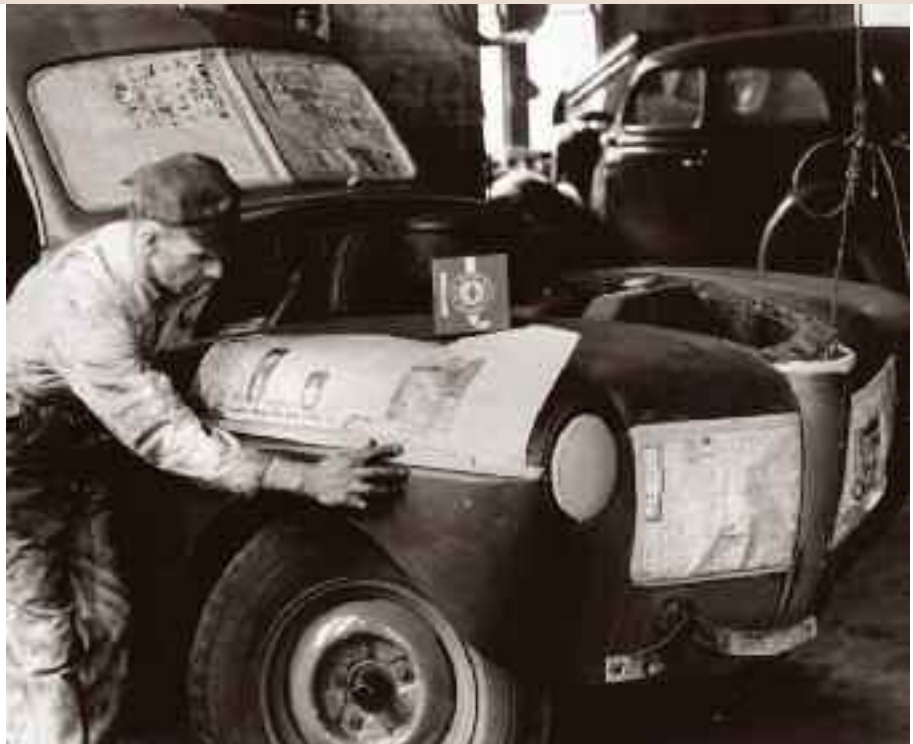
Auto-body worker using Wetordry ™ masking tape, the first reliable masking method for two-tone painting. Its success helped launch the company's tradition of product development for industry needs.
