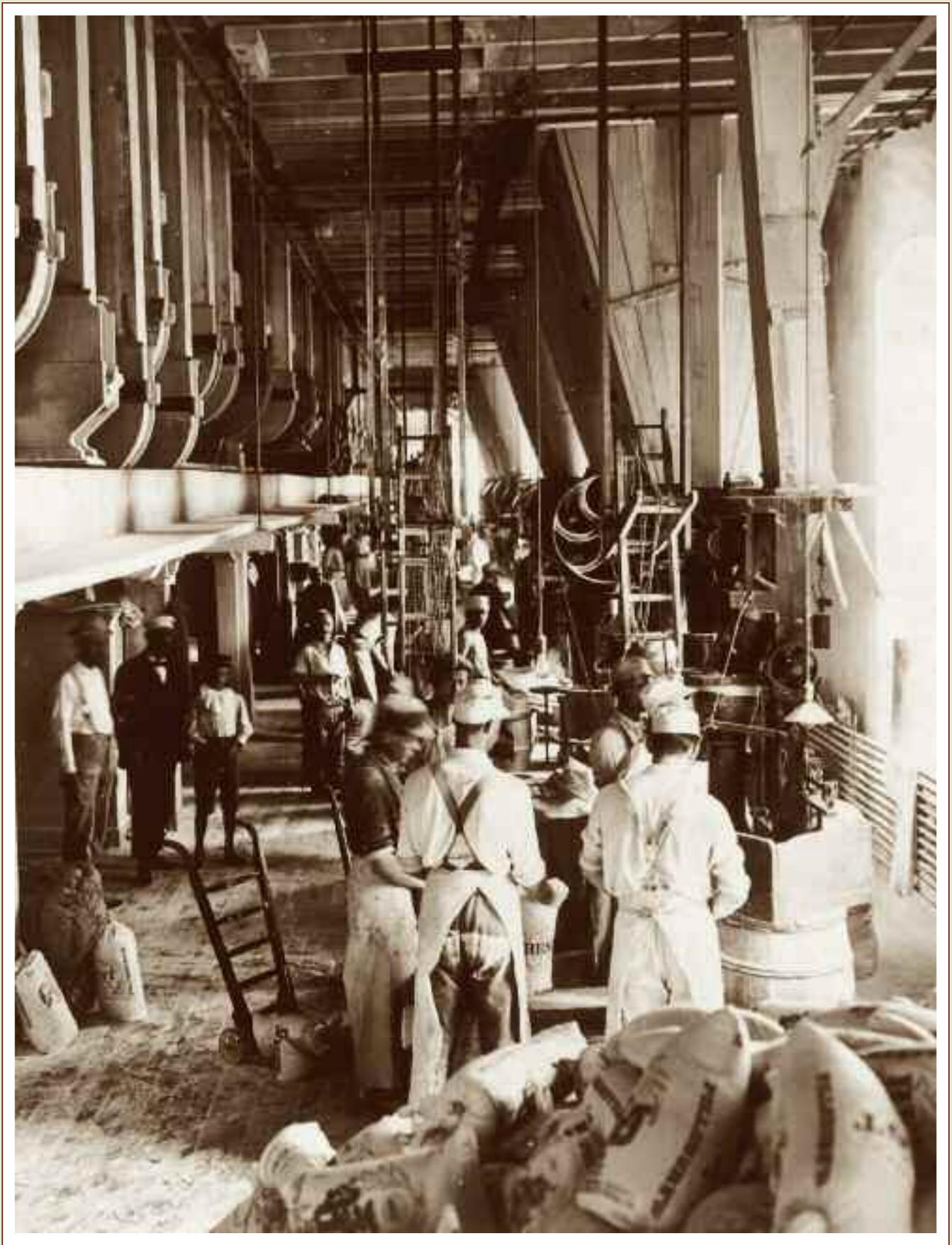
*At the end of the multistage milling process, workers bag and seal flour in the seven-story Pillsbury A Mill, 1902.*
