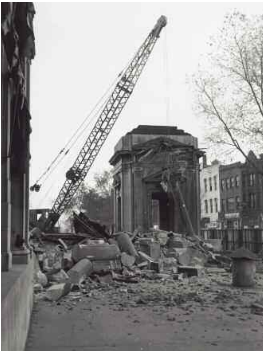
Demolition of the Gateway pavilion, October 1953
