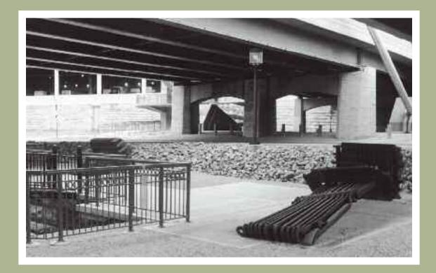
pension bridge and the unfilled tunnel used to place the massive iron anchors for the bridge cables. We even unearthed the bridge anchors and portions of their link bars that attached the supporting cables to the anchors. East-side excavations had to wait for the removal of the deep fill of the existing approach road to the Hennepin Avenue Bridge during construction in 1988. Archaeological monitoring on the east side revealed even more extensive remains of the two early bridges.
