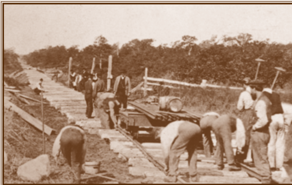
Unidentified work crew laying rails, about 1870
