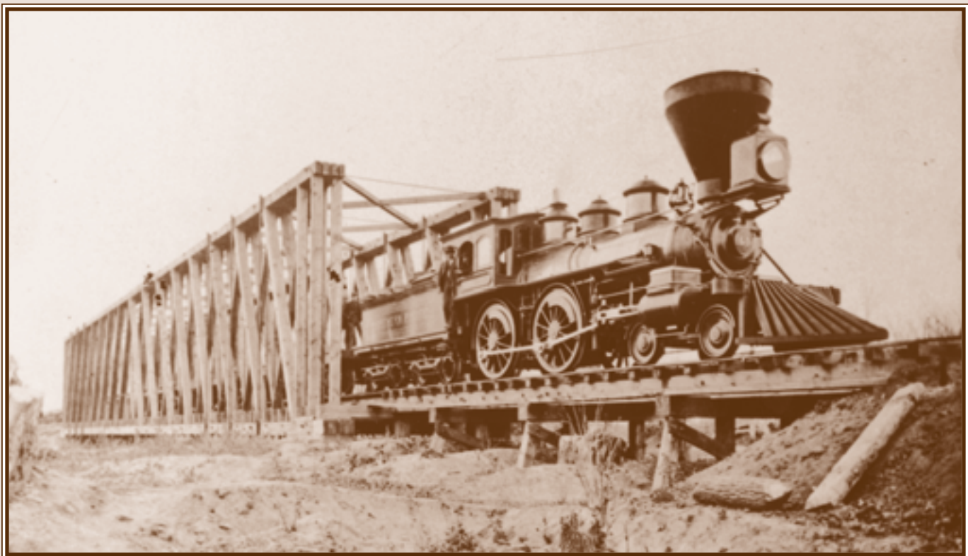
Northern Pacific engine and bridge on the Brainerd line, about 1871
