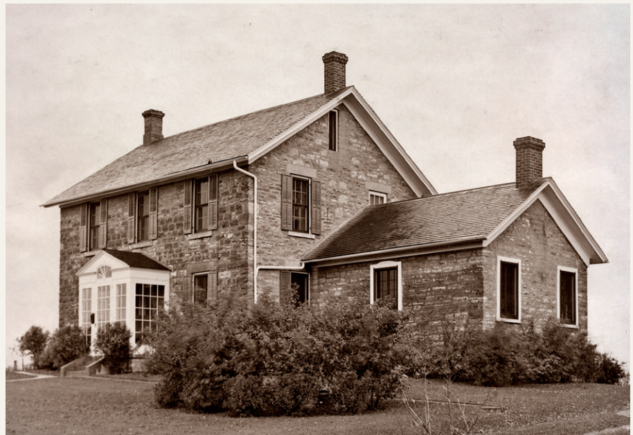
A one-story addition on the north side of the house (date unknown) matches the construction of the main portion of the house except that the lintels and sills at the windows are wood rather than stone. Adjacent to the dining room, this wing originally served as a kitchen—a typical addition for nineteenth-century German American farmhouses. The colonial revival vestibule added later was a typical addition to older houses during the 1920s and 1930s.
