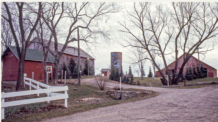
Frederick Spangenberg helped his brother Charles build a granary (right) in about 1875 and a bank barn (back) around 1887. The two-story, gable-roofed granary, which has a lean-to on either side, is constructed with mortise-and-tenon timber framing and sheathed with board and batten. Now demolished, the gable-roofed barn was constructed in a similar manner and sat on a limestone foundation. This photo was taken about 1977.
