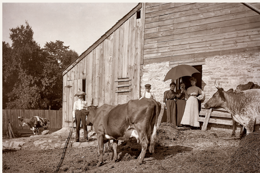
A view of the “bank barn.” At the west end of the barn, livestock could access the lower level on grade. Hay storage on the upper level was accessed from the top of the slope on the other end. Built on a stone foundation, the wood-framed barn was sheathed in vertical wood siding.
