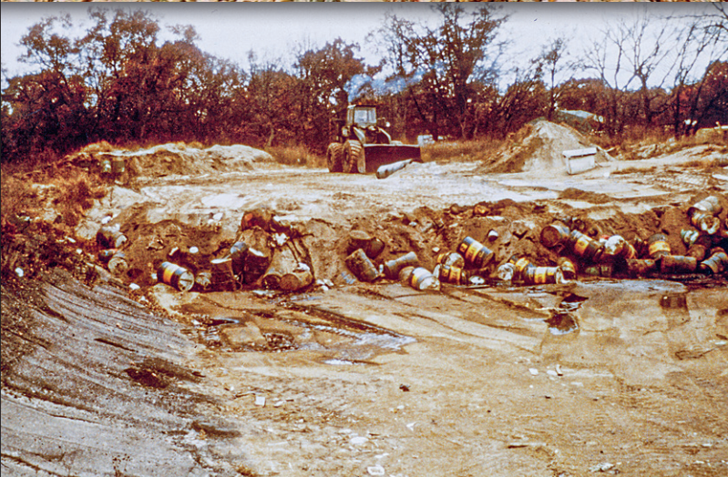
LEFT COLUMN: 1970s disposal of chemical waste into the hazardous waste pit. RIGHT COLUMN, TOP TO BOTTOM: 2019 views: formerly remote landfill now surrounded by development; defining the pit excavation area with shelter tent to protect excavation from weather; excavated drums were placed into the oversized drums seen next to the tent and shipped off-site.
