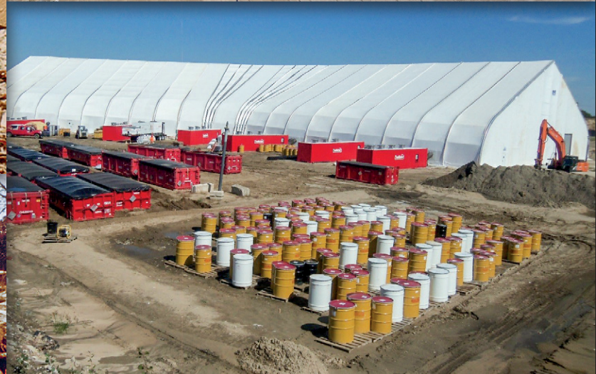
LEFT COLUMN: 1970s disposal of chemical waste into the hazardous waste pit. RIGHT COLUMN, TOP TO BOTTOM: 2019 views: formerly remote landfill now surrounded by development; defining the pit excavation area with shelter tent to protect excavation from weather; excavated drums were placed into the oversized drums seen next to the tent and shipped off-site.
