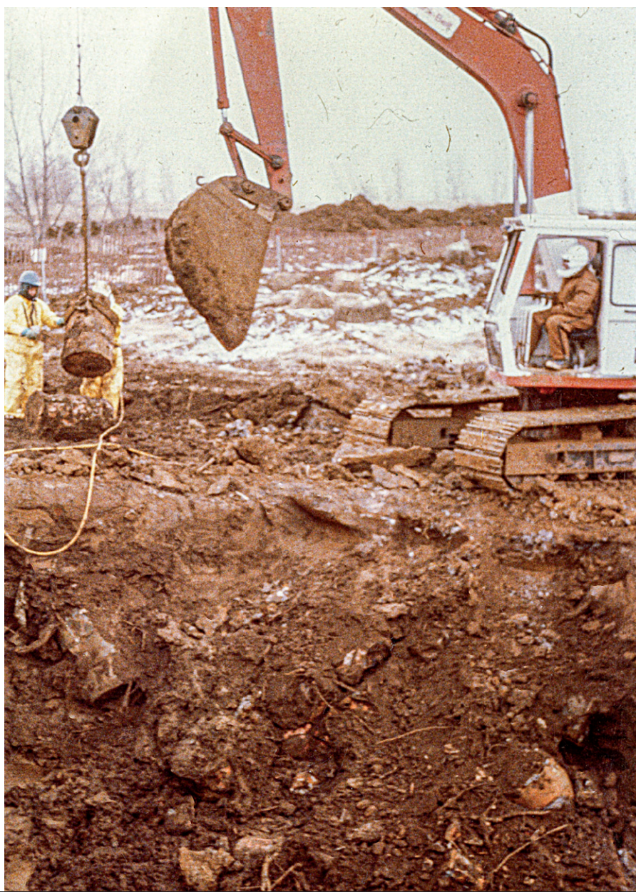
Excavation of drums at Ironwood landfill near Spring Valley, 1970s.
