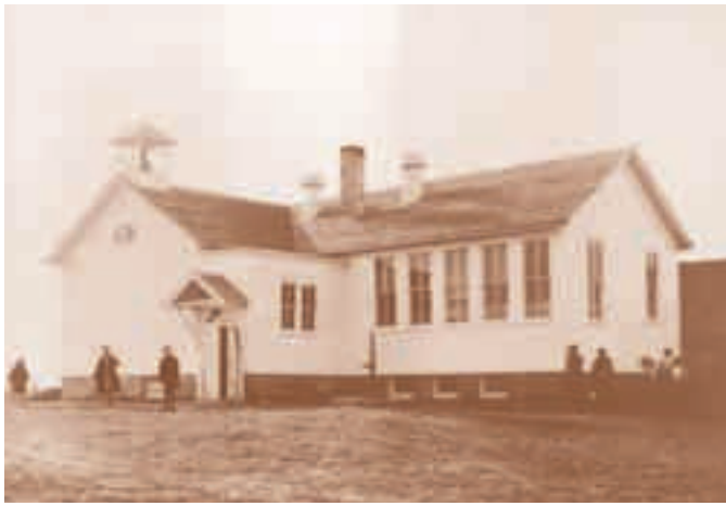
School building in Milo Township, Mille Lacs County, about 1940
