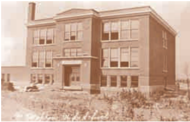
Finishing construction of Wahkon's substantial new school, about 1911. From 1912 to 1937 the facility housed grades one through twelve, including a flourishing cornet band (below).
